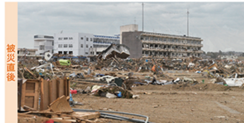
被災直後 Immediately after the disaster 提供: 気仙沼市 Photo credit: Kesenuma City
