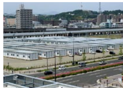
Photo: Temporary emergency housing (prefabricated houses) (Sendai City)
