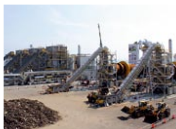
Photo: Secondary temporary scrap yard for disaster waste (Ishinomaki City)
