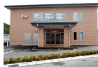
Photo: Restored elder care facility (Ishinomaki City)
