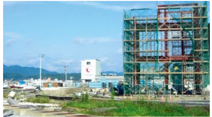
Photo: A fishery processing factory under restoration (Minamisanriku Town)
