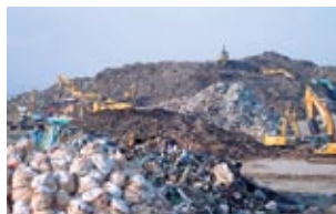
Photo: Primary temporary scrap yard for disaster waste (Natori City)
