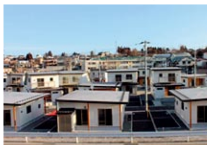
Photo: Public disaster housing (Shiogama City)
