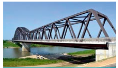
Marumori town (Marumori Bridge)
