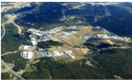
Ohiramura (No. 2 Sendai North Central Industrial Park)
