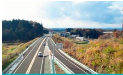
Kurihara city, Tome city (Miyagi Prefecture Northern Freeway)
