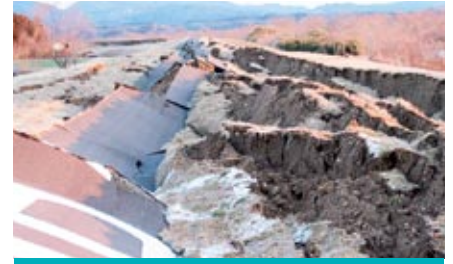
Kakuda city Abukuma river embankment
